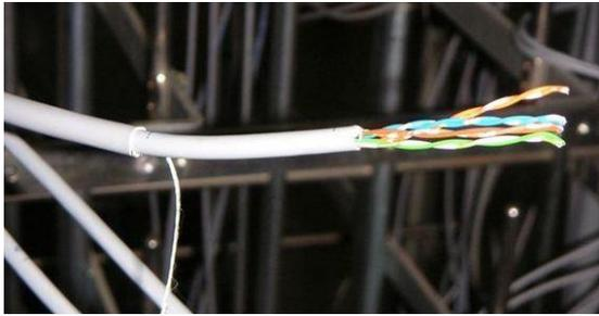
Figura ~~62-64~~ – Sguainatura cavo UTP
